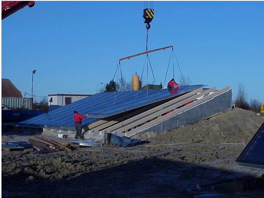
Fig. 2.2.6. Implementation of roof modules (Wagner), Marstal, Denmark [2].
