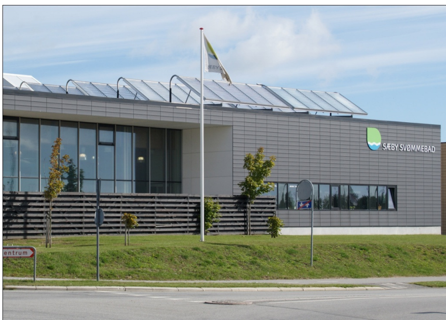
Fig. 2.2.8. Collectors on the roof (ARCON), Denmark [4].
