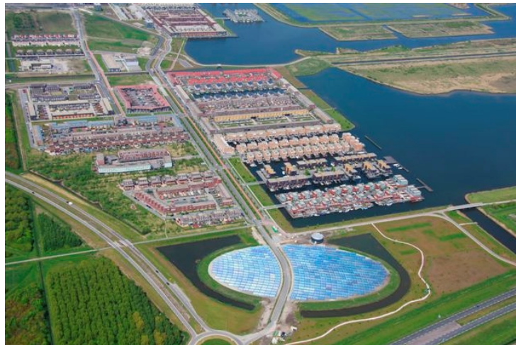
Fig. 2.2.4. "Collector Island" (SUNMARK), Almere, Holland [1].
