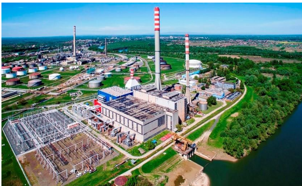
Figure 11: CHP unit in Sisak (Source: https://www.hep.hr/proizvodnja/termoelektrane-1560/termoelektrane-toplane/te-to-sisak/1561 )
