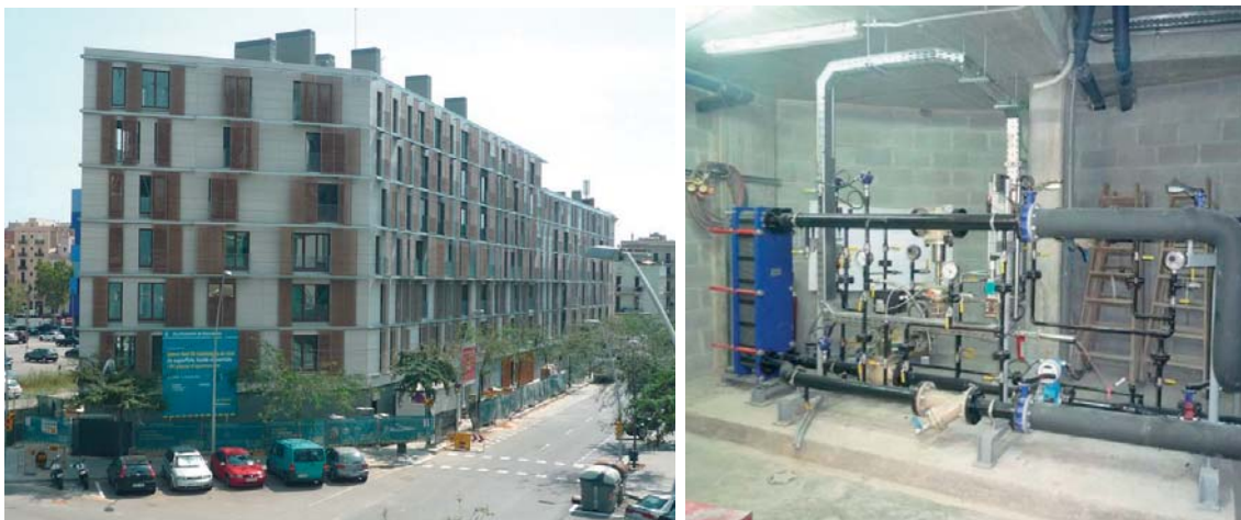
Figure 17: Some 95 apartments connected to district energy in Barcelona Innovation District 22@. (Source: SaAS)
