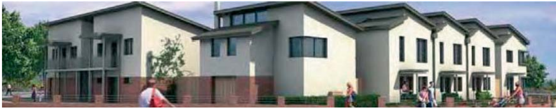
Figure 18: Greenwatt Way development, Slough, UK
